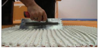
3 Tile can be installed over DITRA-HEAT and DITRA-HEAT-TB immediately. Fill the matting with unmodified thin-set mortar and comb additional mortar over the matting using a trowel that is appropriate for the size of the tile.
