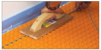
Embed the heating cables between studs, at 3 stud spacing (3-1/2" – 9 cm).
