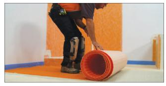
Apply DITRA-HEAT or DITRA-HEAT-TB to the floor, fleece side down. Solidly embed the matting into the mortar.
