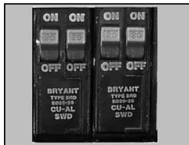
(E) Verify circuit breaker not tripped; if it is tripped, reset it once only.
