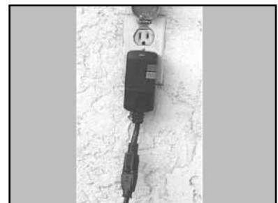
(C) Check to see if the Ground Fault Circuit Interrupter (GFCI) tripped.
