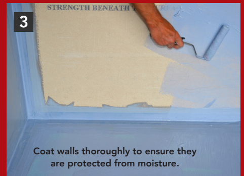
"Tank" the shower base and walls with two full coats of waterproofing.
