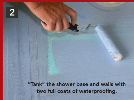
Coat walls thoroughly to ensure they are protected from moisture.
