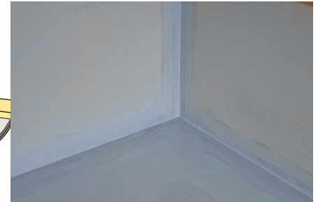
Allow the first full "tanking" coat to dry before topping it with a second full coat.
