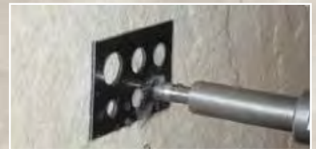
Enter the diamond crown into the hole in the guide pad. Start the water flow and commence drilling
