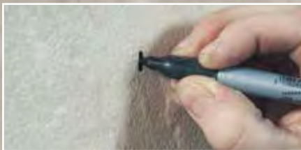
Mark the position of the desired hole
