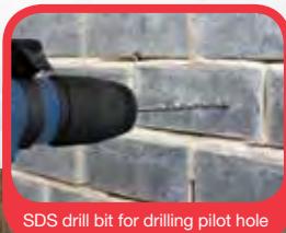
SDS drill bit for drilling pilot hole
