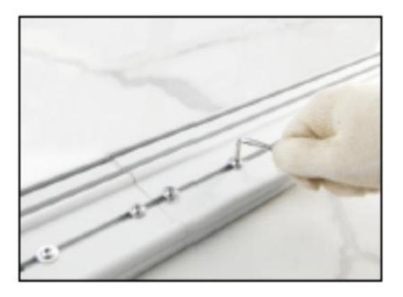
Connecting the guide rails to each other, tighten the screws with a wrench at the connection part.
