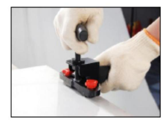
5.Align the center of the clamp with the cutting line and apply increasing pressure on the clamp until the tile snaps along the score line. Use pliers to gently clamp the edges of the tile to help it break off.
