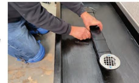
with local plumbing codes. To achieve desired slope/pitch, first use a U-shim which is designed to be combined and stacked with a flat shim as needed. Each U-shim and flat shim are a 1/4" inch thick. When combined together, they provide a total of 1/2 inch of height. Provided the pan is pre-pitched at a 1/4 inch per foot, you can simply place CODA into the pan using U-shims for support if needed; see video.
