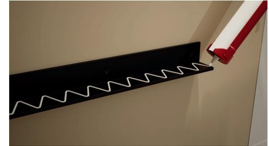
**3 Apply adhesive to the brackets, and then set the bottom board onto the brackets.**
