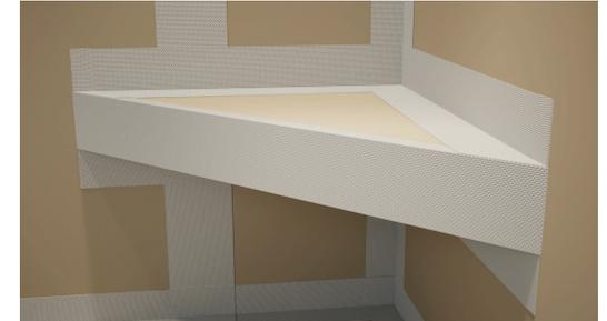
**6. Apply a layer of thin-set and wrap the exposed sides and brackets in provided tape.**
