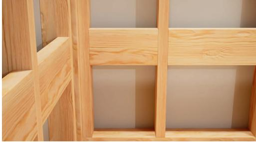
**1. Install blocking at desired height between pre-existing wall studs. Apply wall board according to manufacturer instructions.**
