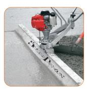
from spot to spot along the screed bar. The back-to-back triangular construction of the ScreeDemon bar is extremely rigid and minimizes variability in the transmission of vibration.
