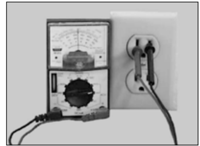
(F) Check power source voltage is 230V - if not 230V, move to another circuit
