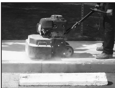
Operate on concrete surface
