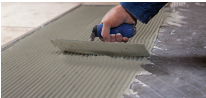
FIGURE 2.21: Install tile/stone flooring
