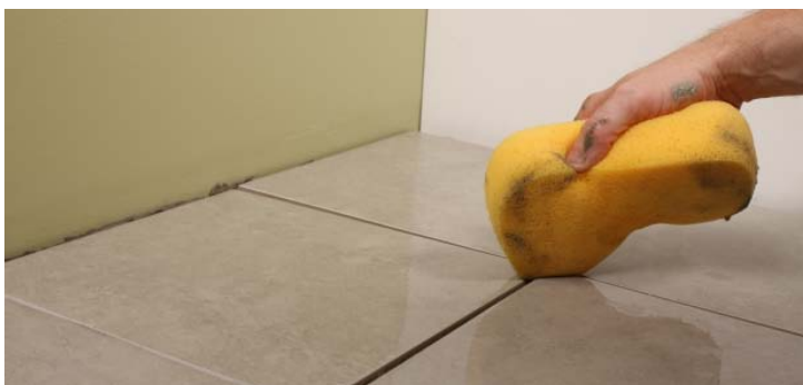
FIGURE 2.23: Clean grout lines
