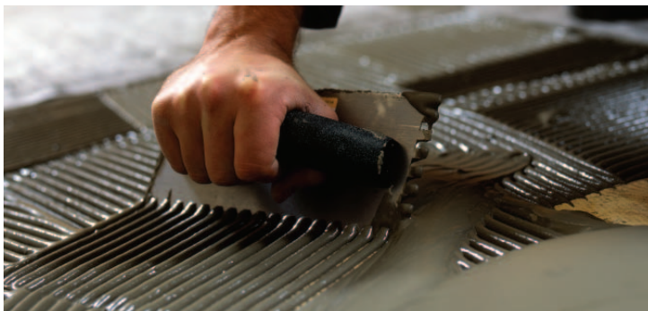
FIGURE 2.12: Spread thinset onto subfloor
