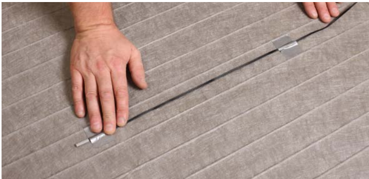
FIGURE 2.16: Secure floor sensor probe
