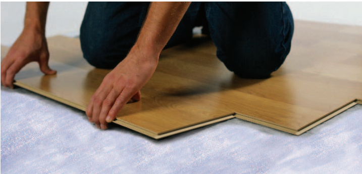
FIGURE 2.33: Install laminate/engineered wood flooring
