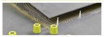
Laying the floor. The size of the tiles, exclusively laid with the "full bed" technique, must be at least 5x5 cm. C2 type adhesive is recommended with a cement type subfloor.
