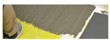
Be sure to level the adhesive and completely fill the cylindrical cavities of the membrane with a smooth trowel and then with a suitable notched trowel.
