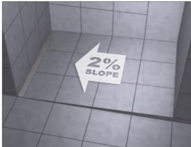
DO NOT DO THIS! This is not an acceptable shower design for an accessible shower. There will be a height difference between the shower floor and the rest of the bathroom floor.
