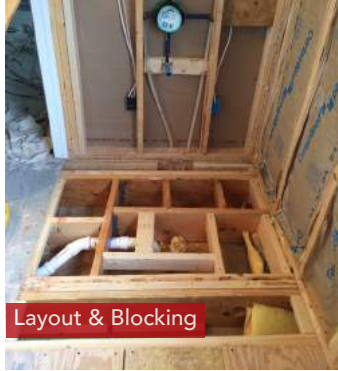
Install Base & Drain
