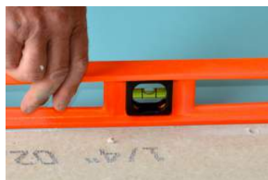
Make sure the shower base is level (bubble centered) all around. Check as you go.
