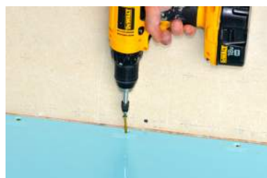
Drive perimeter screws so they are snug, but not so tight as to unlevel the base.
