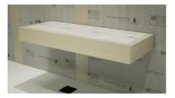
6. Apply a layer of thin-set and wrap the exposed sides and brackets with provided Tape.
