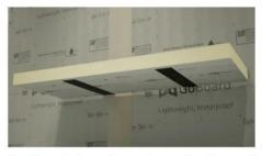
3. Notch brackets into 1st board Apply adhesive to the brackets. Set the board onto the brackets.
